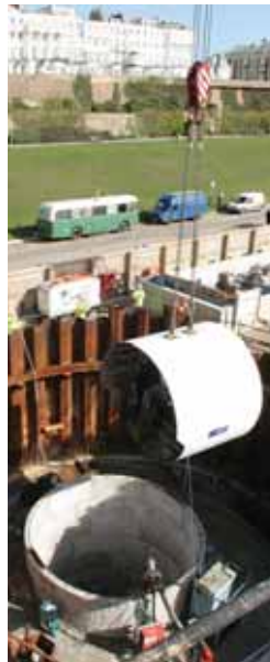
A tunnelling machine being lowered at Black Rock
