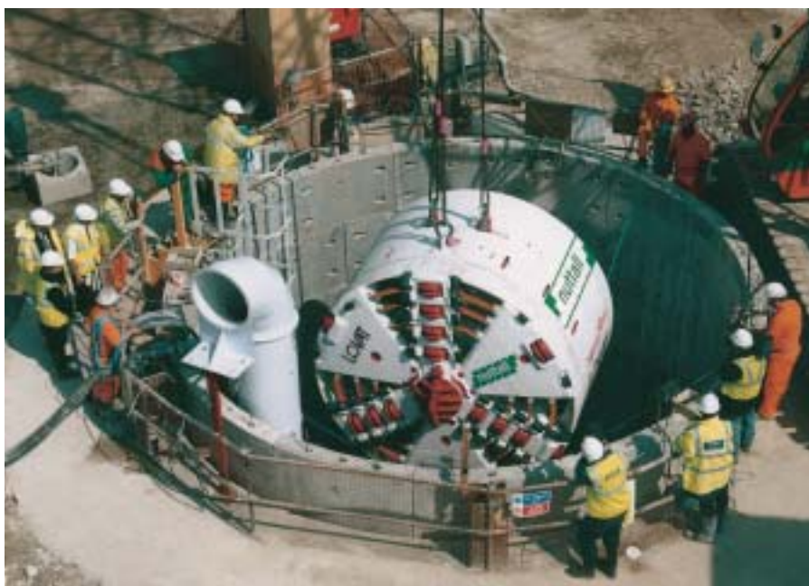
A tunnelling machine, used for a similar scheme in Portsmouth, Hampshire
