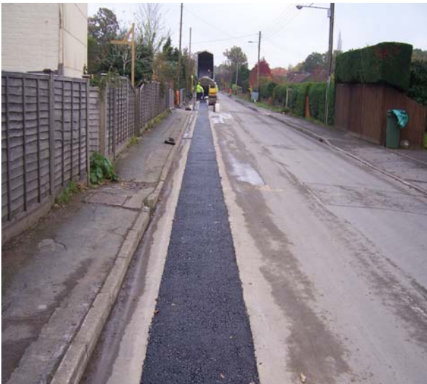
Reinstatement in Church Lane
