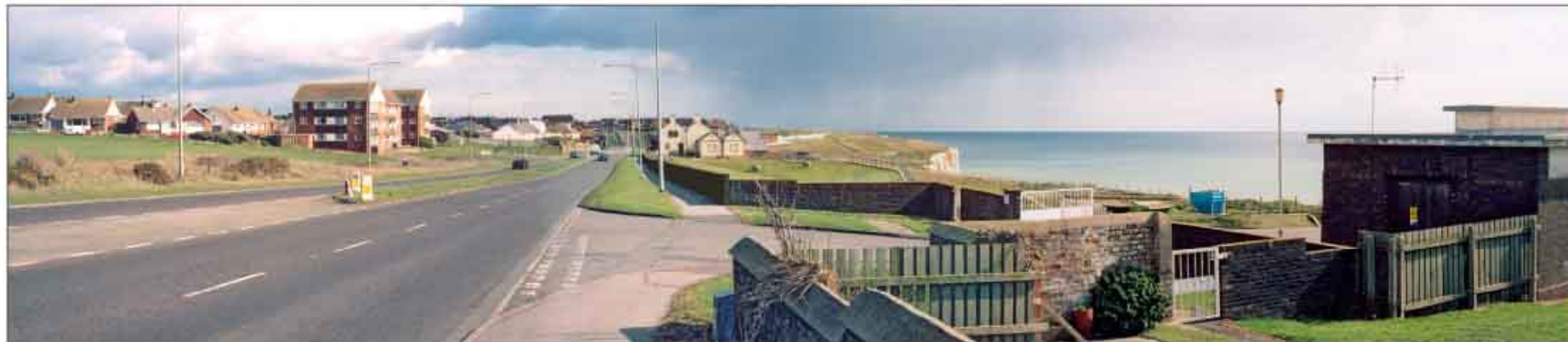
FIGURE 10.4d: the current proposals - with the green roof of the Portobello pumping station visible behind the wall at centre-left
