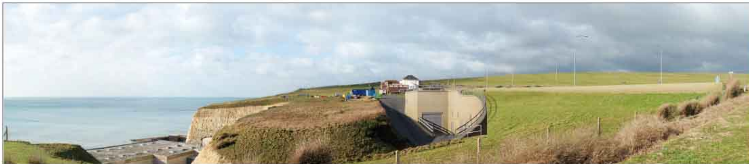
FIGURE 10.4h: the current proposals - showing how the Portobello pumping station would be set into the bank beside Southern Water's existing headworks access road
