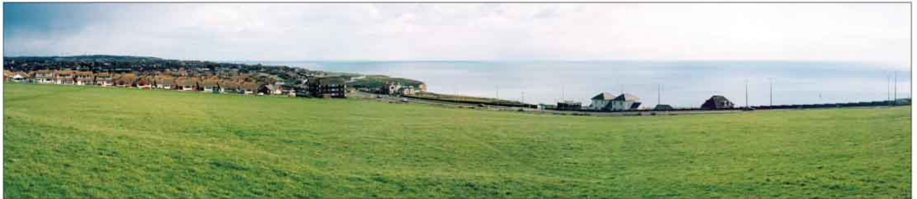
FIGURE 10.4b: the current proposals - photomontage image with the Portobello pumping station in place
