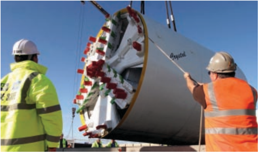
The tunnel-boring machine is lowered into position
