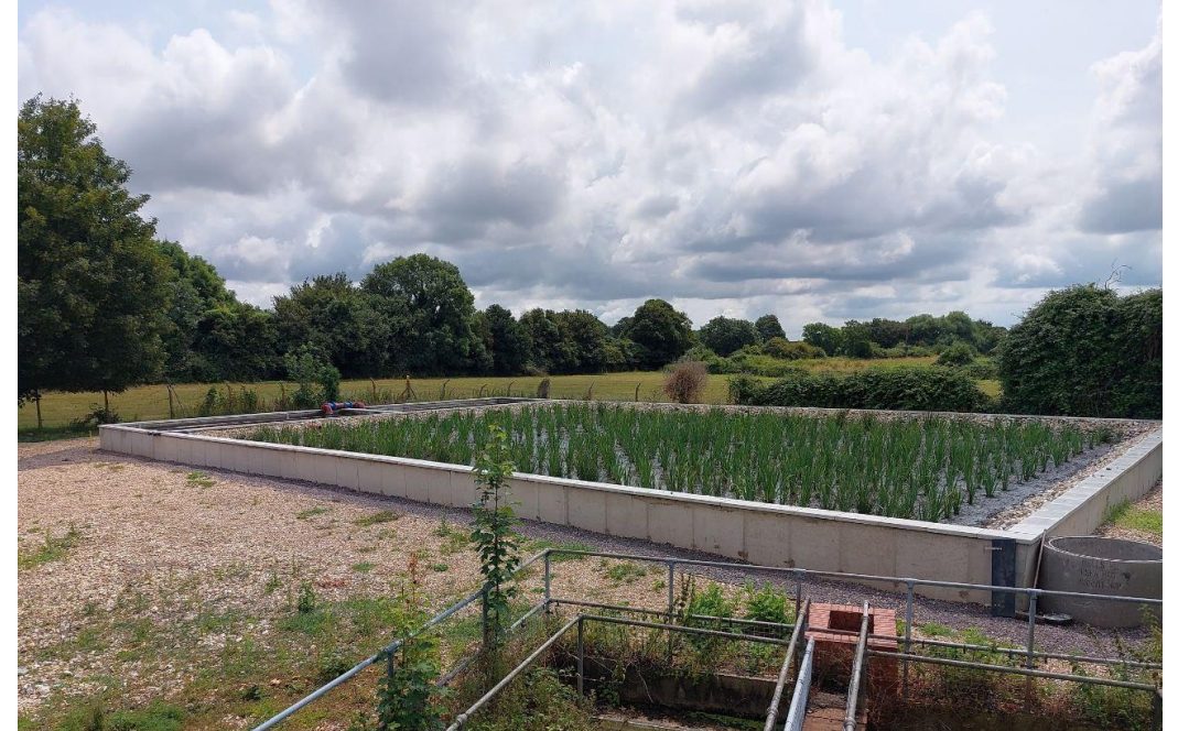
Lavant WTW wetland: using nature to prevent harm from discharges from the storm overflow
