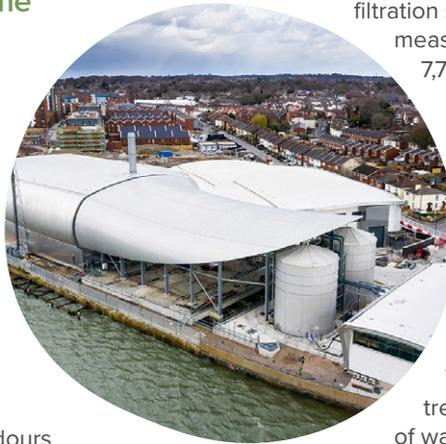
Advanced technologies have also been built into the site, including the largest Membrane Biological Reactor (MBR) in the UK. This is a filtration system of membranes that measure a total length of more than 7,700 kilometres.
