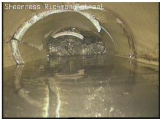
Richmond Street, Sheerness. Extensive survey of a complicated network has revealed collapses and fractures with large amounts of infiltration.
