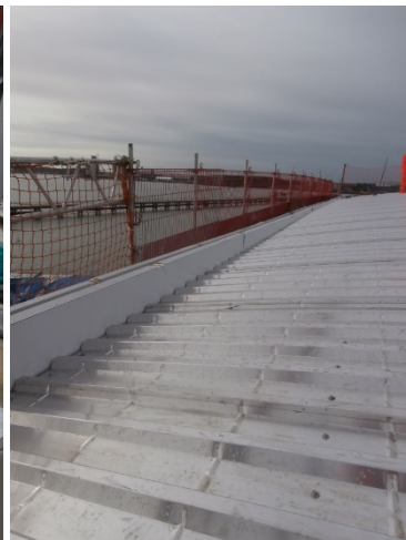
First roof-cladding layer
