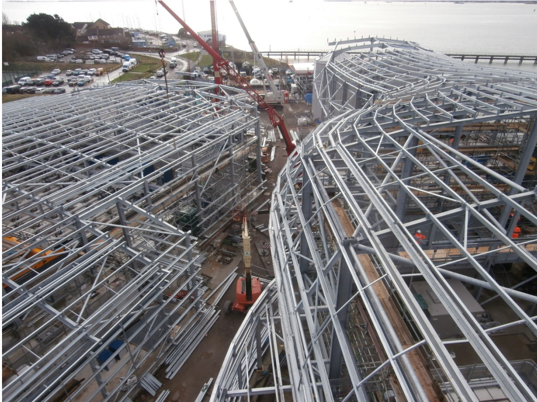
Superstructures of the primary and secondary buildings
