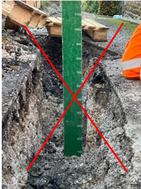
Figure 6: Not approved photo of trench depth
