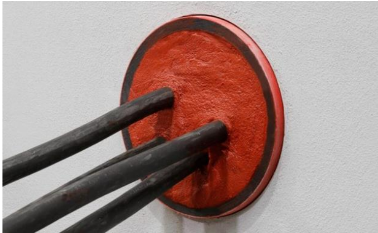
Figure 15: Picture of use of approved sealing product
