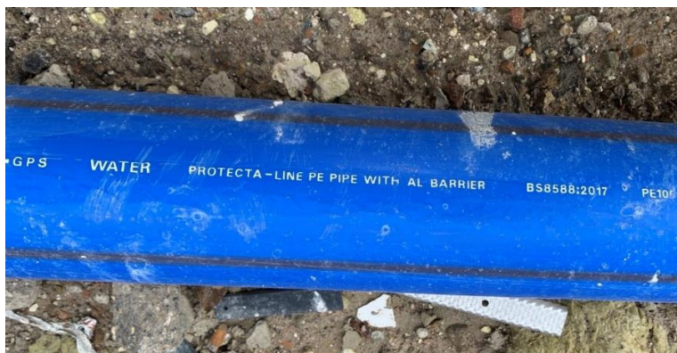
Figure 20: Approved photo showing an example of barrier pipe
