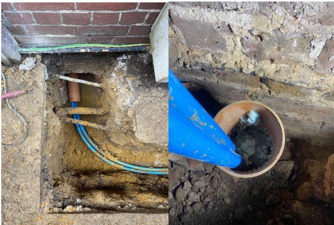
Figure 13: Approved photo of duct entering property Figure 14: Approved photo of pipe in sealed duct
