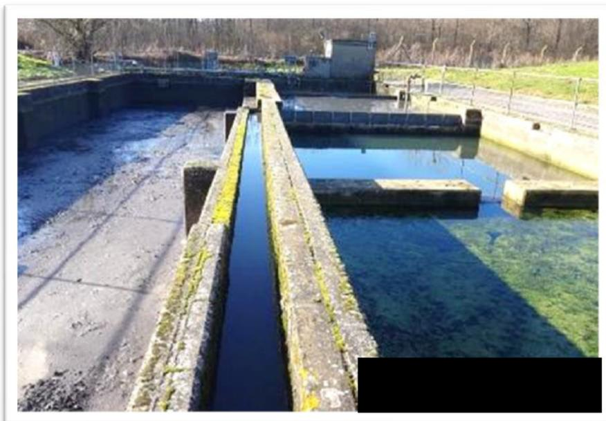
**Figure 21: Solid material in storm tank**
