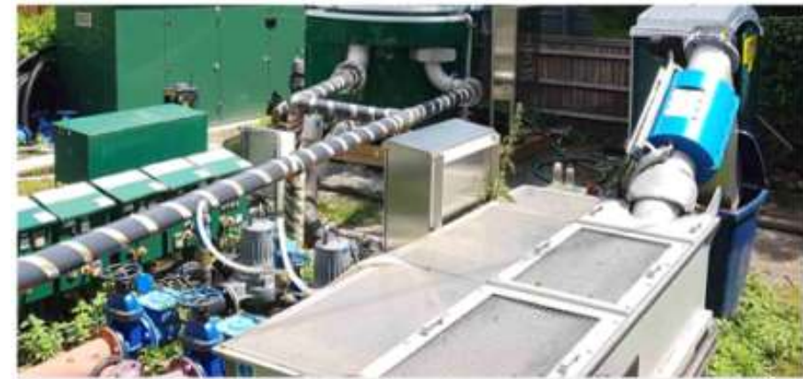
Photo of groundwater treatment unit.
