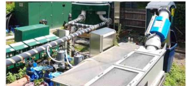
Photo of groundwater treatment unit.
