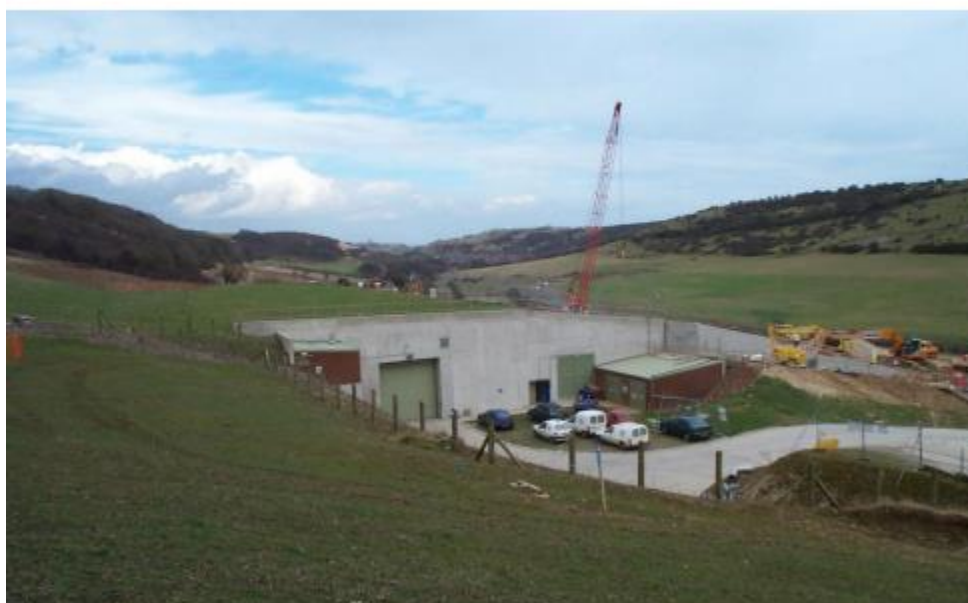
Photo 2.1: Broomfield Bank underground WTW 4
