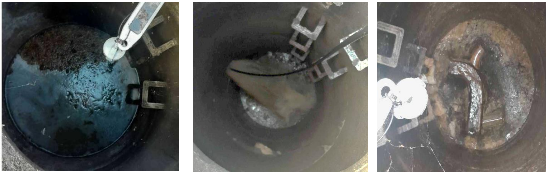
Figure 16 Surcharged manhole prior, during and after jetting
