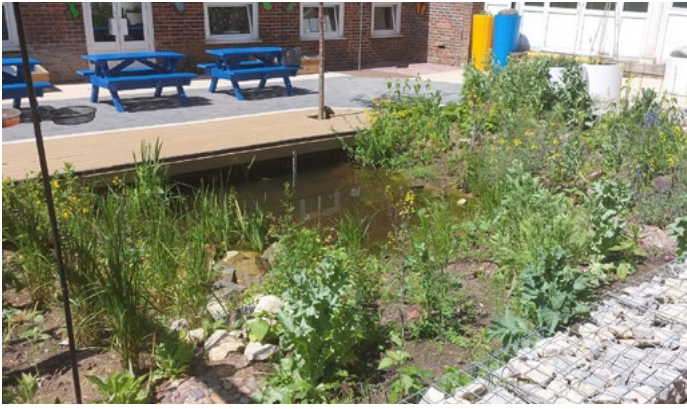
▲ Raingarden installed in Brighton
