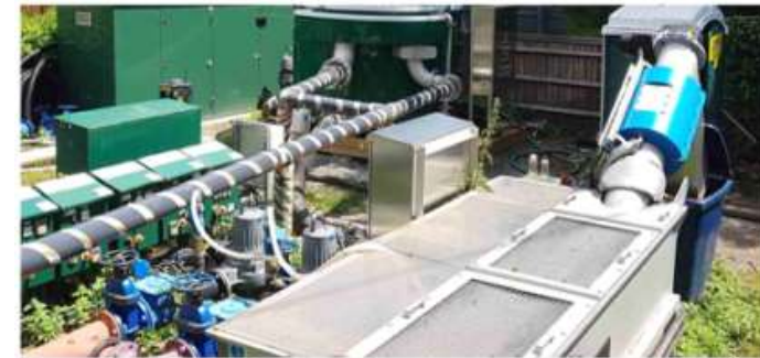
Photo of groundwater treatment unit.
