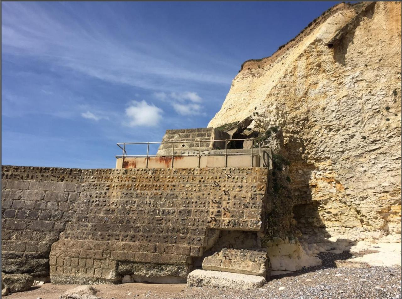
The groyne requires stabilisation, the supporting wall on the eastern groyne has deteriorated significantly as shown in Figures 6 and 7<sup>24</sup>
