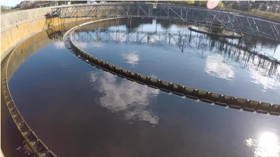
Figure 8 Image of secondary settlement tank at Peel Common and source for the water recycling pilot plant
