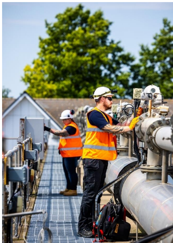
Weatherlees Hill Water Treatment Works
