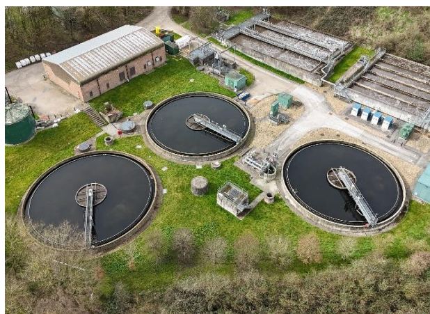
Centralised system - Morestead Road WTW
