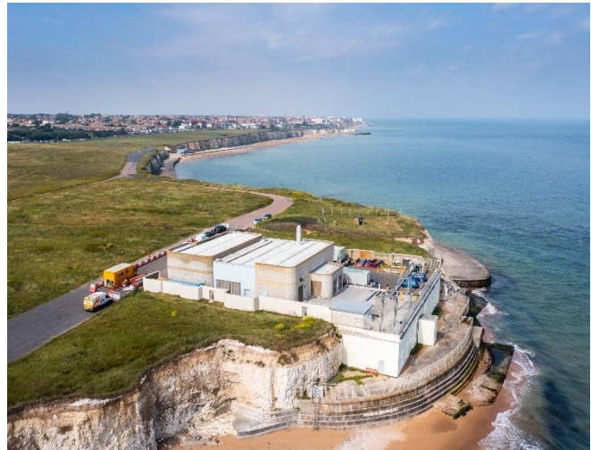
Margate Wastewater Pumping Station
