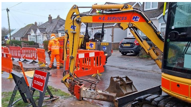
Emsworth sewer separation works
