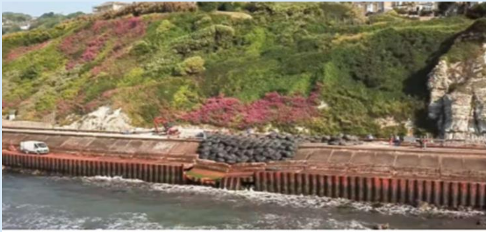
Figure 3: Eastern Esplanade, Ventnor – Emergency Work (December 2022)
