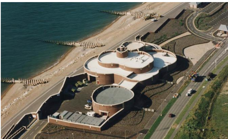
Figure 1: Eastbourne Wastewater Treatment Works predominantly located underground
