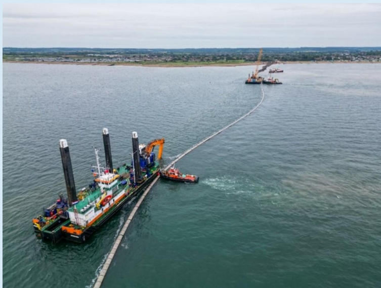
Figure 2: Sea-outfall replacement at Swalecliffe
