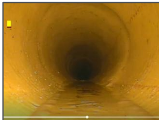
The same sewer after sealing
