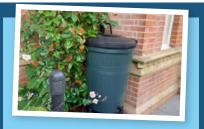
184 properties in Havenstreet offered a slow-drain water butt to trial whether it reduces storm overflows from pumping station at bottom of village which activates whenever there is 5mm of rain in 12hr period.
