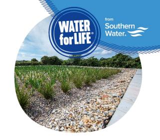
We're using constructed wetlands as an eco-friendly alternative to storm tanks, to help reduce storm overflows and as part of the sewage treatment process. Water is treated by a variety of physical, chemical, and biological processes, such as sedimentation, filtration, precipitation, adsorption, plant uptake and microbial decomposition.
