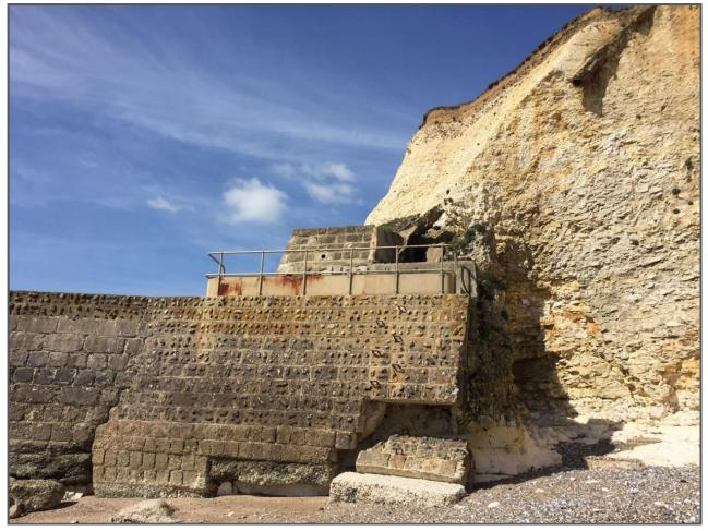
The groynes require stabilisation, the supporting wall on the eastern groynes has deteriorated significantly as shown in Figures 6 and 7<sup>24</sup>
